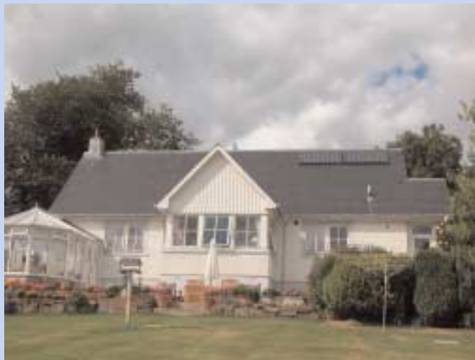
Fig 1: Solar water heating system installed in Perthshire home with the help of an Energy Saving Trust household grant.
