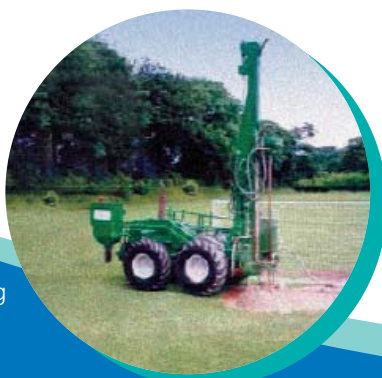
Typical drilling rig
